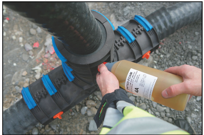
Clip Shell & joint foaming
