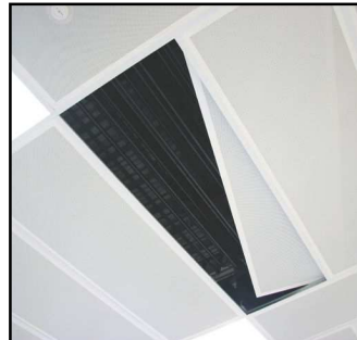
"Radiant" Passive Chilled Beam above Ceiling
