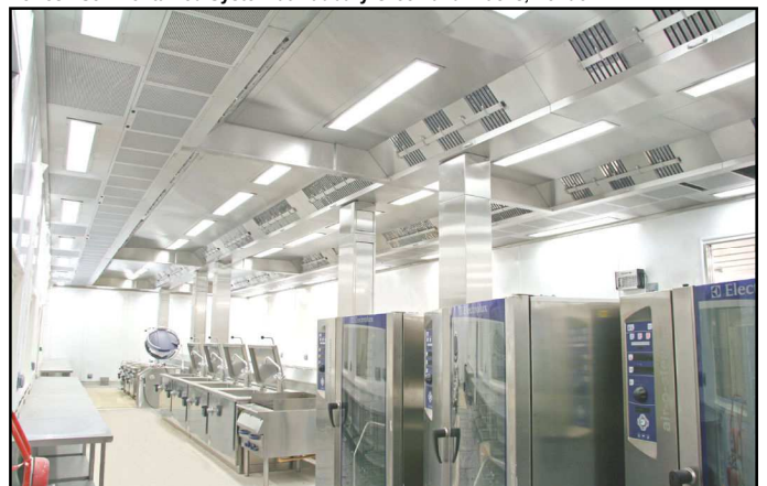
Silverline Ceiling Installed at HMP Parkhurst, Isle of Wight
