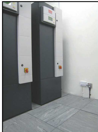
Refrigerant gas detection within a server room from high level cassettes or down blow ACUs
