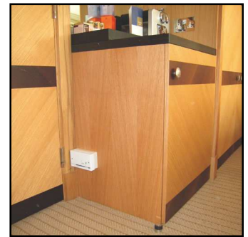
Apartment & hotel room refrigerant gas detection
