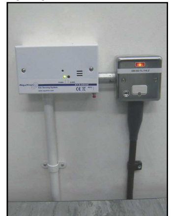
Refrigerant gas detection within a server room from high level cassettes or down blow ACUs
